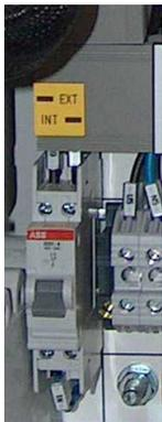
In order to put the remote panel in operation, there is a specific switch inside the control box marked “INT - EXT” . This switch must be turned to "ext".
